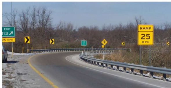
Figure 4: Roadside barriers, chevron signs and speed limit sign
