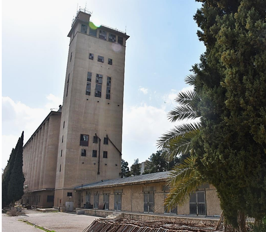
Figure 12. Hafezieh Grain silo (by Narges Rasm, 2024)
