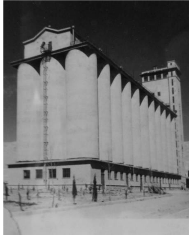
Figure 13. Hafezieh Grain Silo (Mahdiun, 2018)
