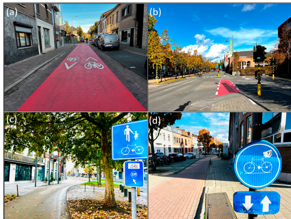
Figure 2. Examples of bicycle infrastructure facilities in Hasselt. (a) bicycle-prioritized street paved in red, (b) separate bicycle traffic signals at a junction, (c) shared bicycle lane with pedestrians, separated from motorized traffic by trees, (d) bicycle lane separated from motorized traffic by a median.
