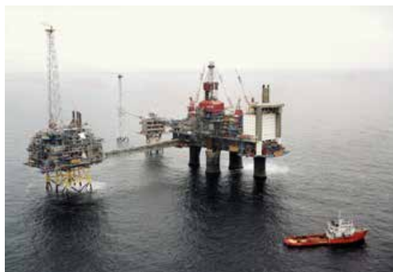
Fig. 23. Sleipner gas-field platform of Statoil, Norway. The installation CO 2 -rich natural gas is produced from this platform and re-injects the stripped CO 2 into sandstone-layers beneath the gas reservoir © Statoil.
