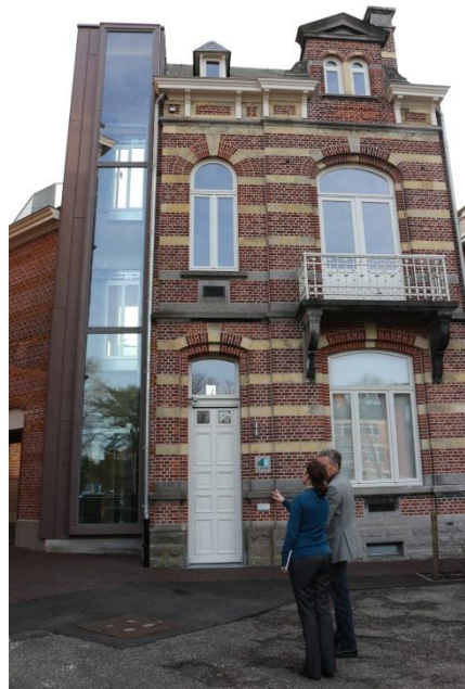
Figure 5. Facade renovated porter's lodge
