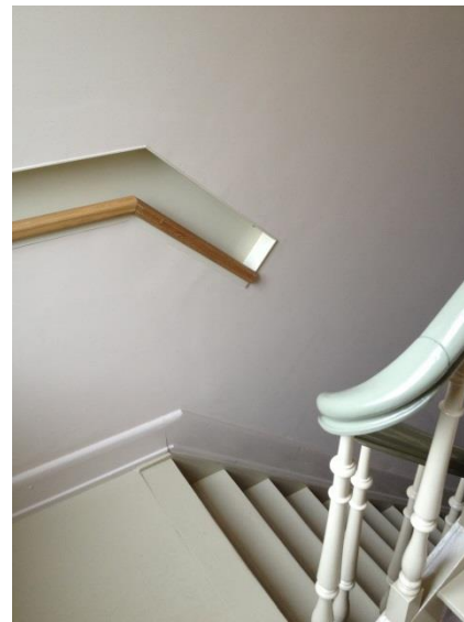
Figure2. built hand rail (right).
