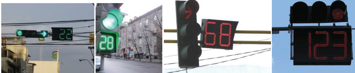
Figure 1 Examples of numerical countdown timers installed at traffic lights. They are used for both counting down the green and red phase.
