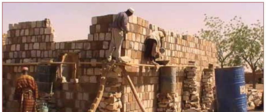
Bouw hulppost in Nalou.
