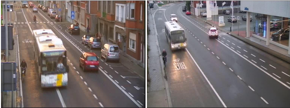
Figure 1 – Observation sites: Kortrijk (left) (3.1m wide - in line with guidelines) and Ghent (right) (4.2m wide – not in line with guidelines).
