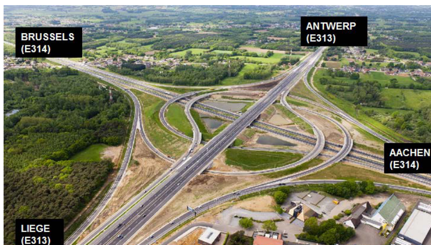
Fig. 1. Freeway interchange E313-E314 in Lummen, Belgium.
