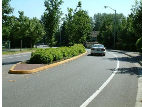
Figure 30 Gate constructions with wider traffic lanes and recovery area ('Transportation Resources - Neighborhood Traffic Calming - Medians', 2011)
