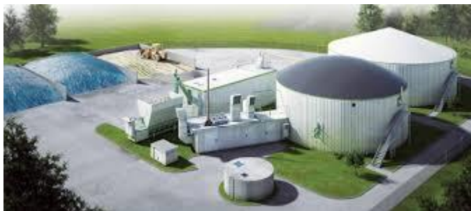
Figuur 19: Vergistingsinstallatie (Viessmann)
