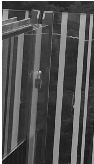
Figure 12: Bolted connection between beam and column
