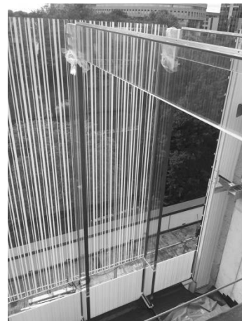
Figure 25: Beam-Column-Pane-Connection structure
