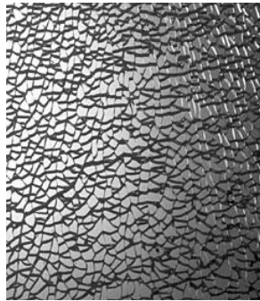
Figure 5: Breakage pattern toughened glass
