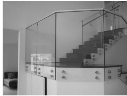
Figure 2: Application of a secondary structural glass element as a balustrade
