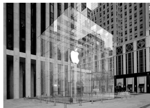
Figure 4: Construction entirely out of structural glass components
