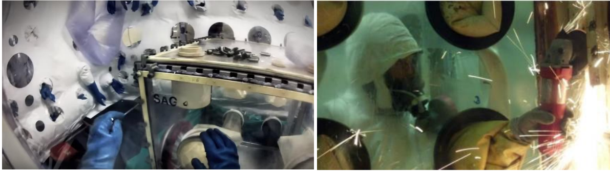
Figure 34: glove box dismantling in a glove tent [61]
