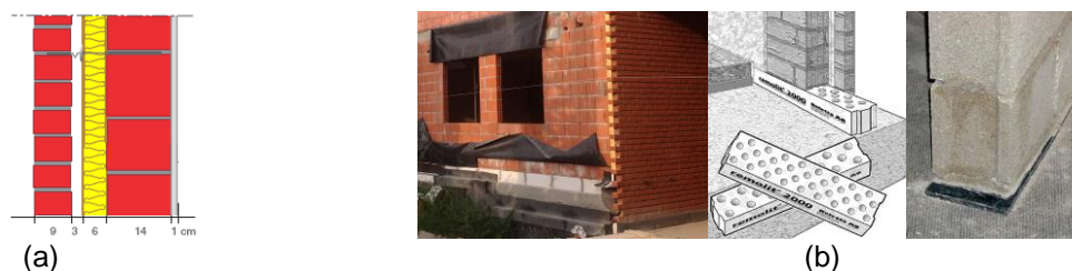
Figure 1. (a) Configuration of a masonry wall in Belgium ; (b) Thermal cut with AAC blocks (left) or foamglass (middle) and acoustic cut with rubber (left)
