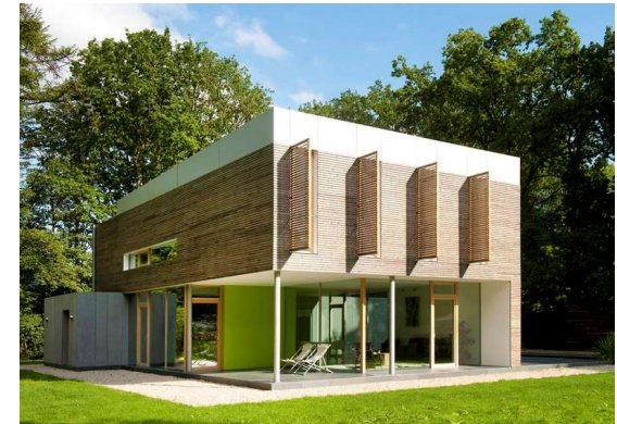
Single family house in Kalmthout (B) by Eprojecten
