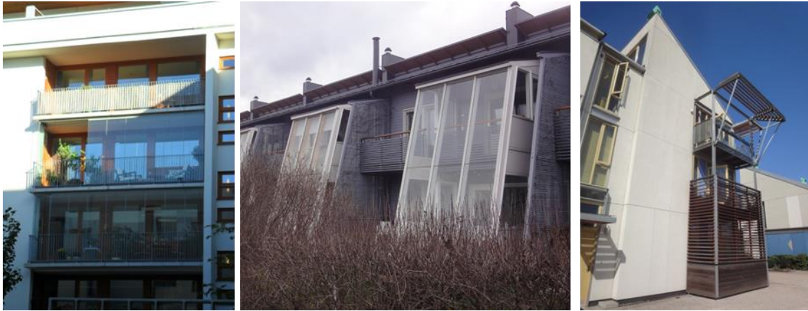
Figure 1: Pictures of some listed individual measures: {glazed balcony} (left, 'BO-01' in Malmö, Sweden), {microclimatic space} (middle, 'Eco-Viikki' in Helsinki, Finland), and {sun-protection louvres} (right, 'GMV II', London, UK). (photo by Bart Janssens, 2012)
