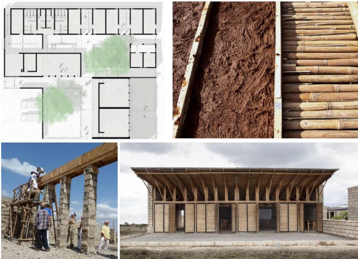
Figure 2: Example of a Design & Build project / Live Project, conducted in Nairobi by students of the Technical University of Munich (TUM), Germany: from design, over testing and prototypes to construction and use. (source: Faculty of Architecture TUM)
