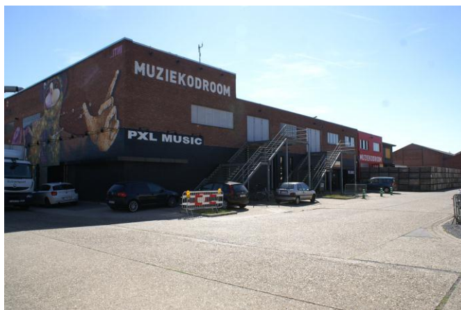
Figure 3 – The retrofitted slaughterhouse, now a concert hall and rock academy (Hippo architecten)
