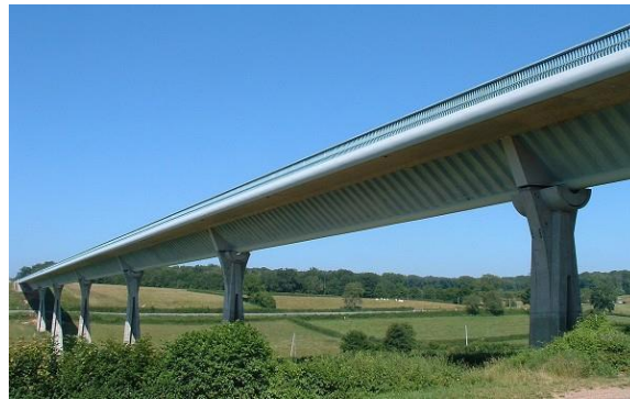
Figure 4: Val de Maupre Viaduct [24] p.1
