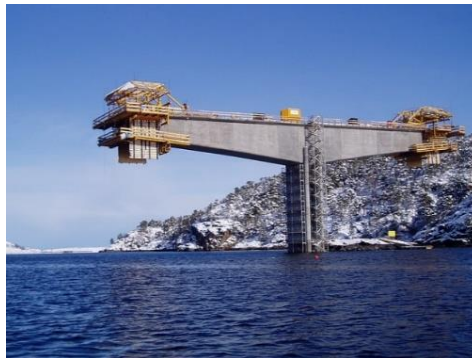
Figure 11: Execution example cantilever construction technique [27]
