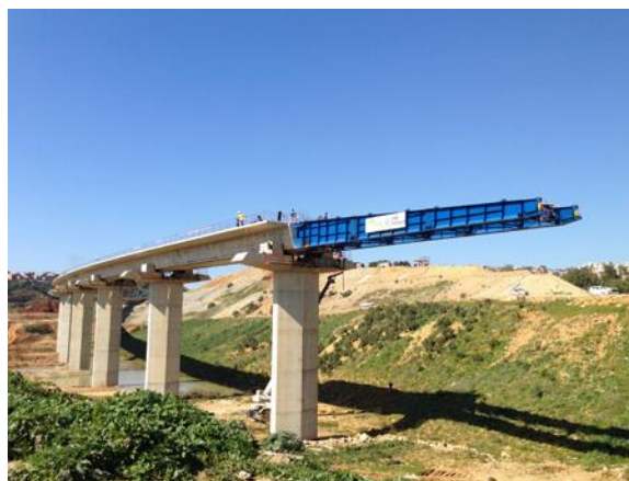
Figure 9: Execution example incremental launching method [25]
