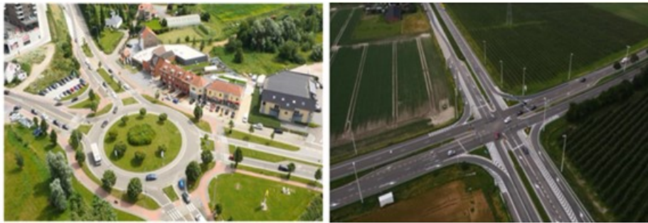
Figure 4.4: The data collection sites: UAV view of the roundabout (left-side); UAV view of the signalized intersection (right-side).
