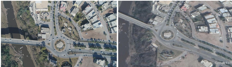
Figure 7.2: The studied roundabout at Location 1; image from the UAV (left-side); Google earth satellite image (right-side)
