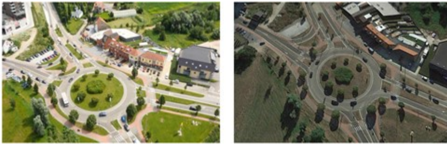
Figure 6.2: The UAV view of the studied roundabout (left-side); and Google Earth satellite image of the roundabout(right-side)
