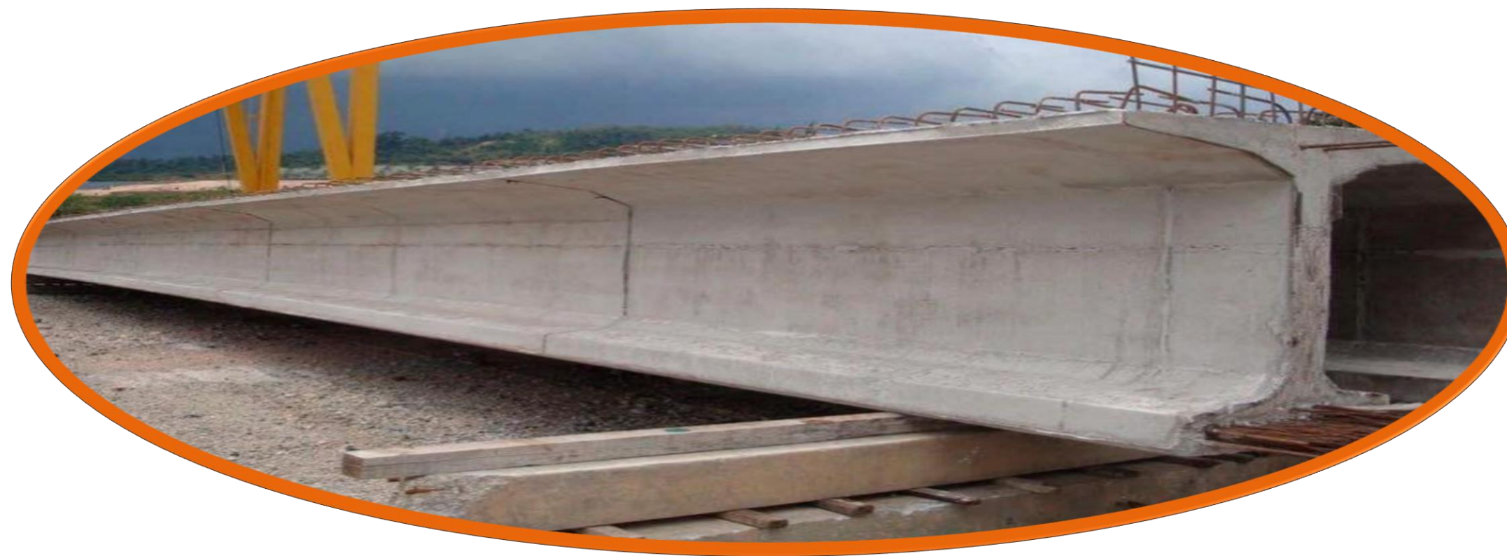
Figure 1: Prestressed I-girder [1]
