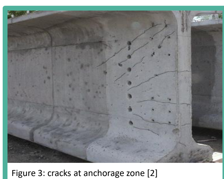
Figure 3: cracks at anchorage zone [2]
