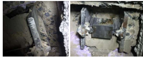
Fig. 14. Bottom view, slide of steel profile, Cv2.
