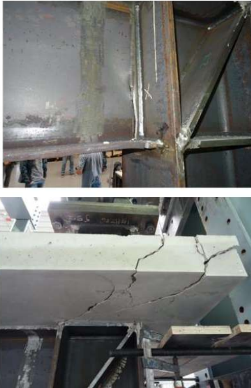
Fig. 4. Observed damage at failure.
