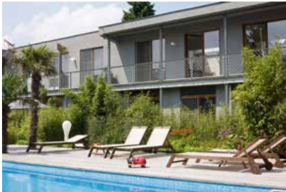
FIG. 16-18: OLD FACTORY SITE, ANTWERP. B-ARCHITECTS.
