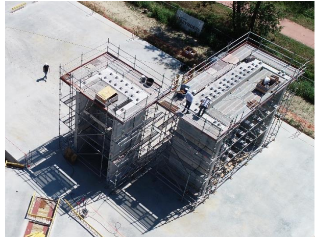
Figure 3: Reaction floor and walls after prestressing
