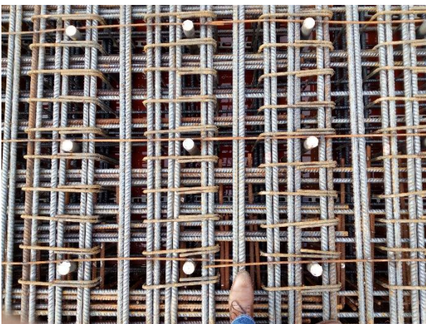
Figure 2: Reaction floor reinforcement lay-out and anchor point grid.
