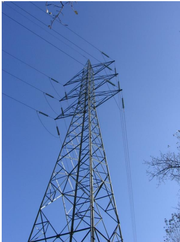
Figure 8: 150kV transmission tower build at Keerbergen [17]
