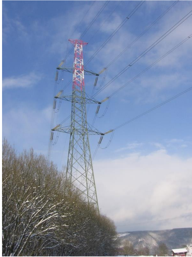
Figure 7: 380kV transmission tower build at Brume [17]
