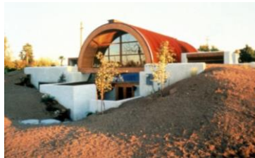
Figure 25: House in Tempe, Arizona, uses earth-sheltered construction methods to help decrease cooling costs. Photo by Pamm McFadden [26]
