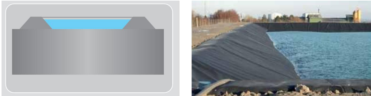
Figure 23: Left: schematic sketch of a water pond heat storage. Right: a 75 000 m 3 water pond under construction at Marstal solar heating plant [23]
