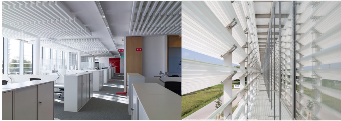
177 Figure 3 (left), overview of the façade with the automated louvers opened; Figure 3 (right) Exterior – Windows 178 Double-skin façade combining glass louvres made of extra-clear glass (outside skin) with super-insulating 179 glazing and white spandrel double glazing (inside skin); Architect: Philippe SAMYN and PARTNERS sprl, 180 architects and engineers – BEAI sa, Photographer: Jean-Michel Byl, Courtesy Notice: AGC Glass Building - © 181 Project : Philippe SAMYN and PARTNERS sprl, architects and engineers – BEAI sa [33] 182
