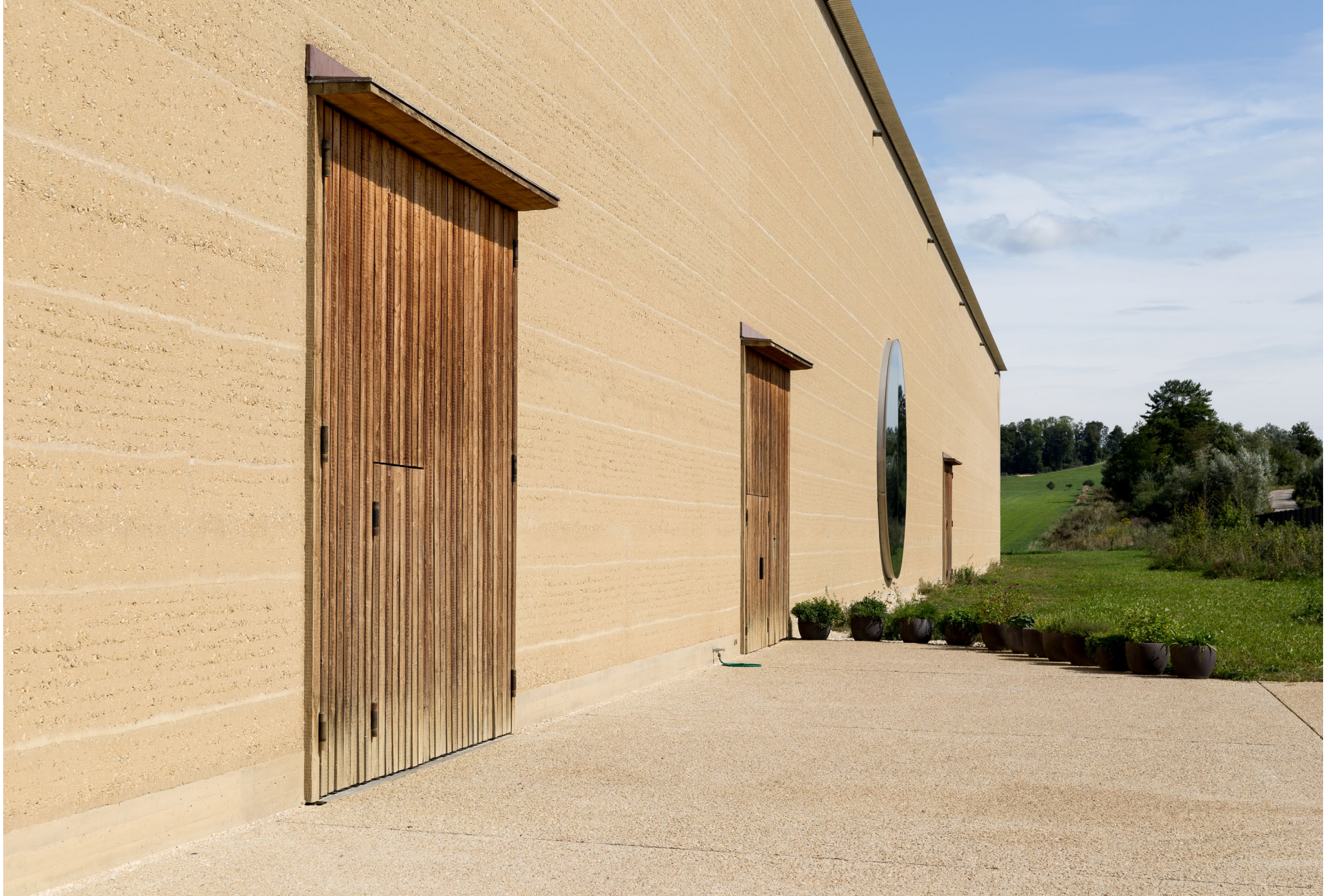
Ricola herb center, rammed earth - Martin Rauch architect: Herzog & De Meuron image: Jasper Van der Linden, 2019
