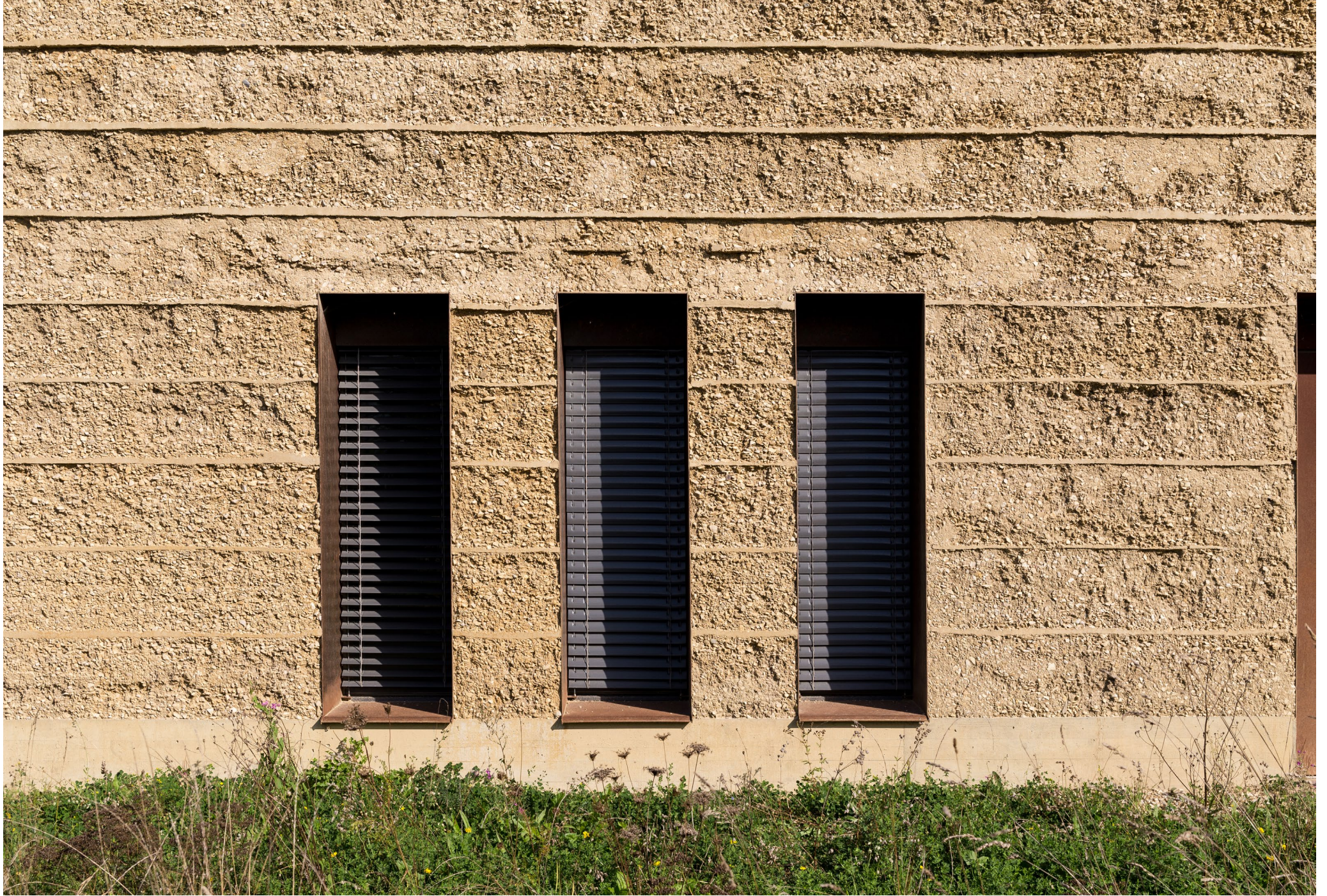
swiss ornithological institute, rammed earth - Martin Rauch architect: :MLZD image: Jasper Van der Linden, 2019
