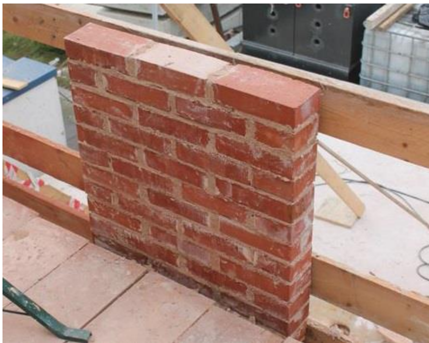
Figure 15: Parapet on the South building façade [4, p. 9]
