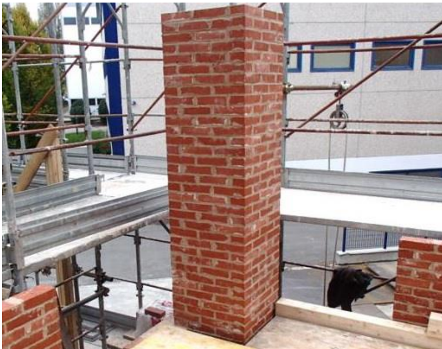
Figure 13: Slender chimney at the South-West corner of the building [4, p. 9]
