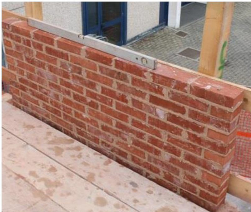
Figure 17: Parapet wall on the East building façade [4, p. 9]
