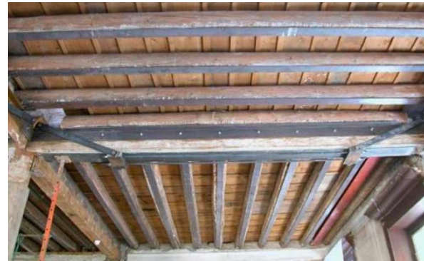
Figure 8 Strengthening of timber using steel by conversion into truss girder (left) and increasing cross section (right) [9]
