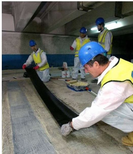
Figure 9 Application of FRP reinforcement on-site from a roll of unhardened fabric [13]
