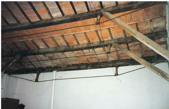
Figure 8 Strengthening of timber using steel by conversion into truss girder (left) and increasing cross section (right) [9]
