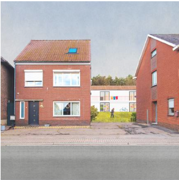
Park City [14] View of the block from road with new terraced houses in the back
