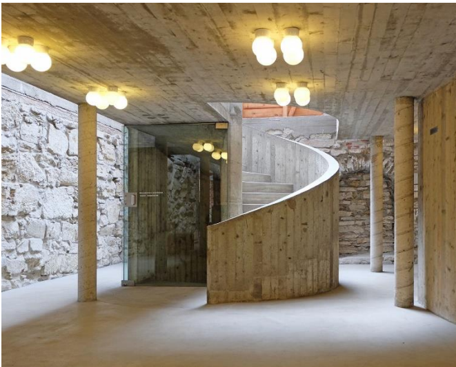
FIGURE 8 THE NEW CONCRETE RAMP CONNECTS LIGHTLY TO THE EXISTING BASE ON SMALL CONCRETE COLUMNS (SVERRE FEHN - HEDMARK MUSEUM HAMAR, N.D.)
