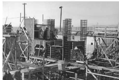
FIGURE 45 THE BOILER STRUCTURES UNDER CONSTRUCTION (BURLINGTON ELECTRIC DEPARTMENT ARCHIVE, 1952-1976)
