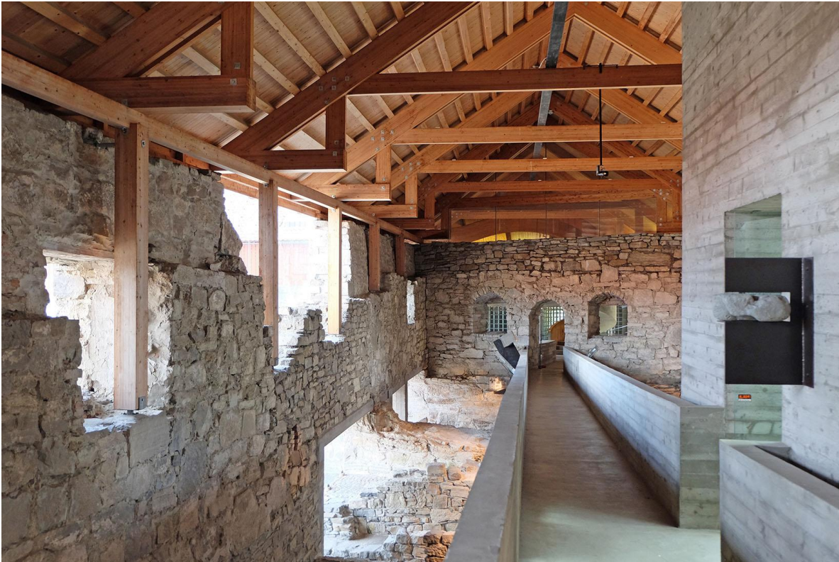
FIGURE 6 FEHN USED MATERIALITY TO DISPLAY THE DIFFERENT LAYERS (SVERRE FEHN - HEDMARK MUSEUM HAMAR, N.D.)
