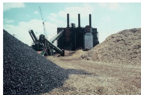
FIGURE 46 THE MORAN PLANT DURING THE WOODCHIP CONVERSION (MORAN PLANT 1954-1986, N.D.)
