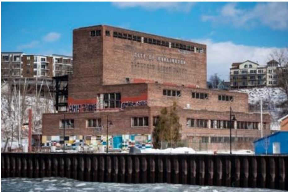
FIGURE 58 VIEW OF THE PLANT FROM THE LAKE. PHOTO BY GLENN RUSSELL FOR VTDIGGER (ASCH, 2020)
