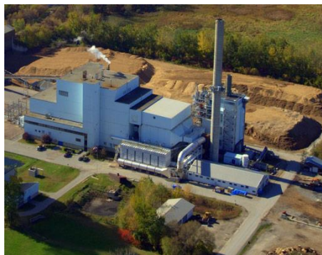
FIGURE 47 THE McNEIL WOOD-POWERED ELECTRIC GENERATING FACILITY (BURLINGTON ELECTRIC DEPARTMENT, N.D.)
