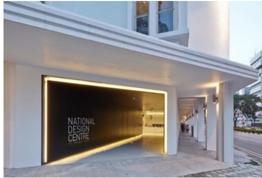
IMAGE 40 NATIONAL DESIGN CENTRE MAIN ENTRANCE
