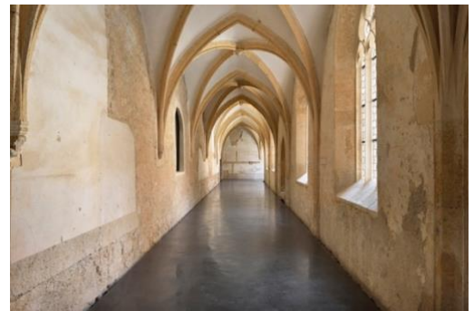
IMAGE 37 CONCRETE FLOOR ON MONASTERY HALLS
