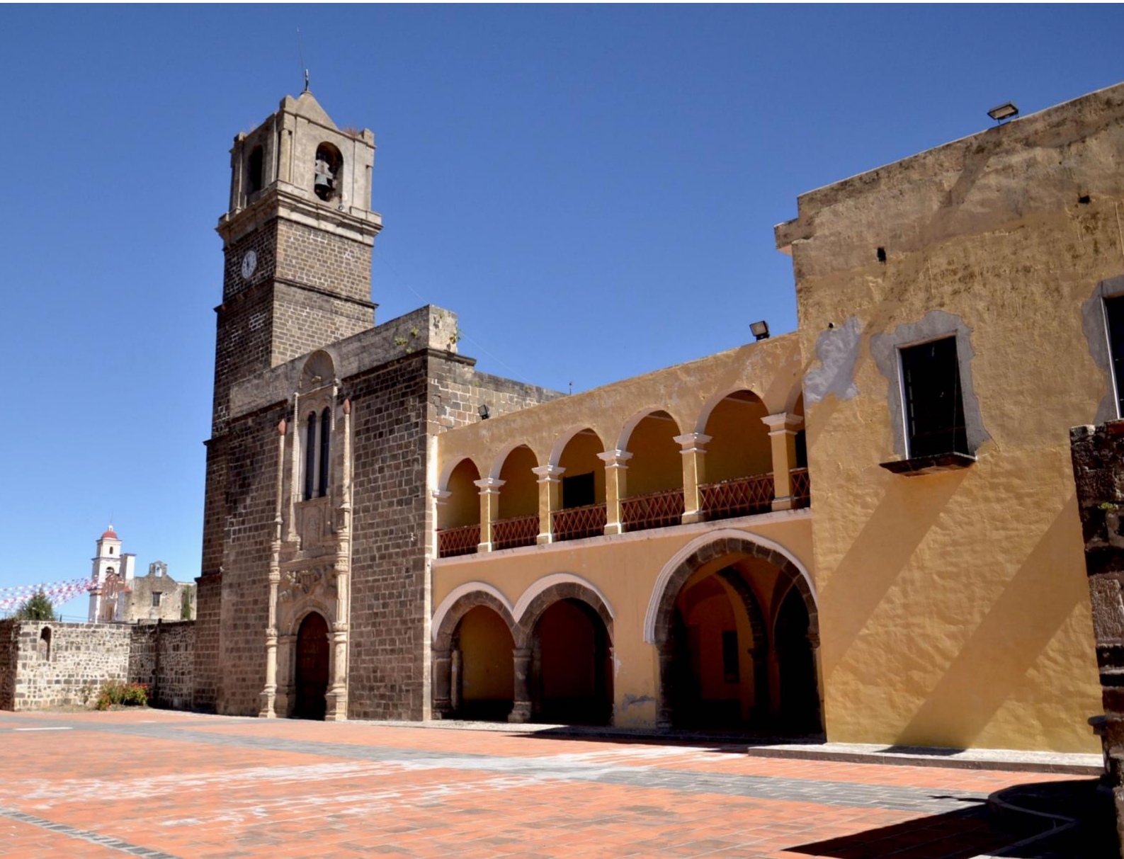
IMAGE 1.MAIN FACADE SAN ANDRES CALPAN MONASTERY
