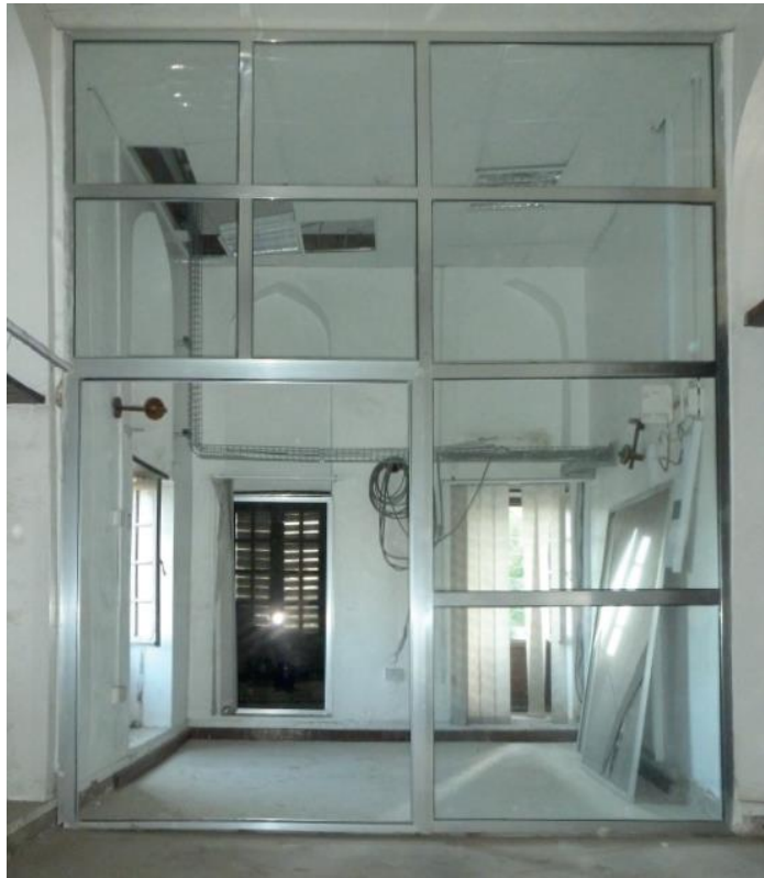
Fig 14: Old Boma before restoration
