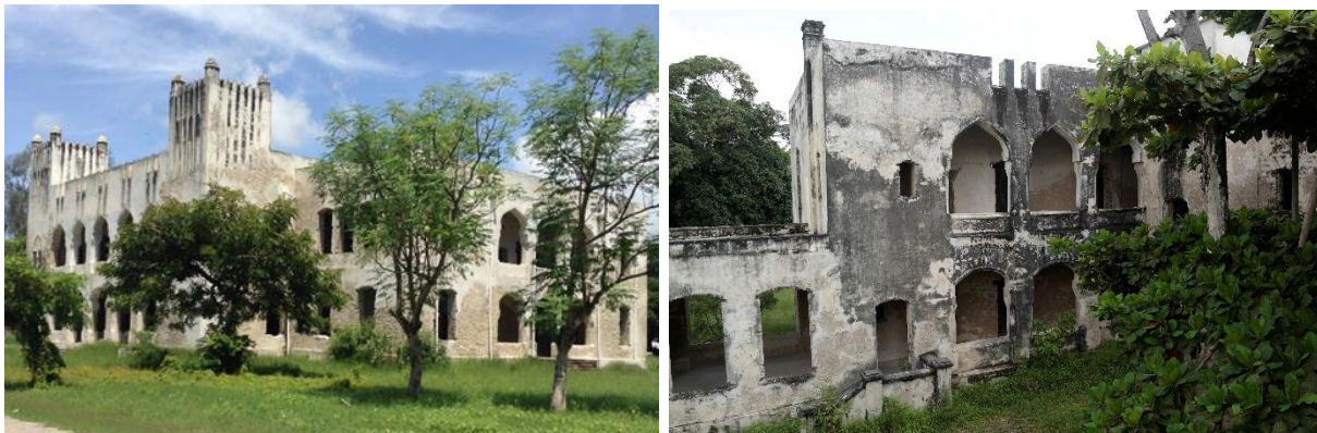
Fig 5: Recent pictures of the old Boma building
