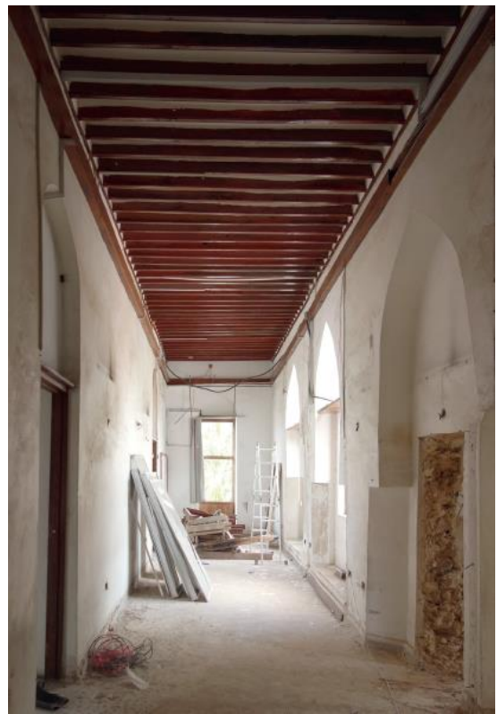
Fig 15: Old Boma during restoration
