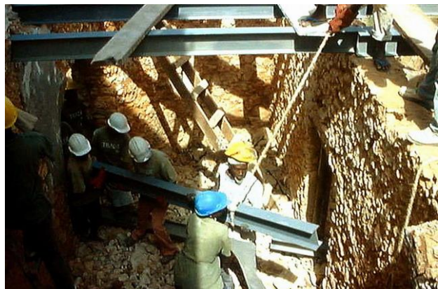
Fig 22: Replacing the I-beams
