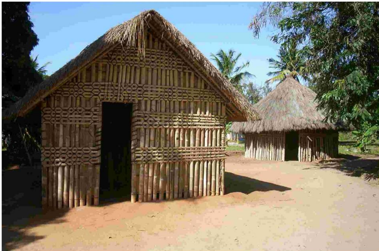
Fig 39: A typical Nyakyusa bamboo house
