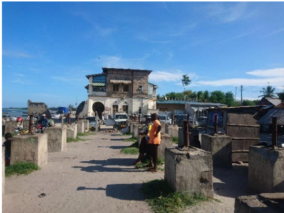
Fig 42: Footings on which Usagara store house stood
