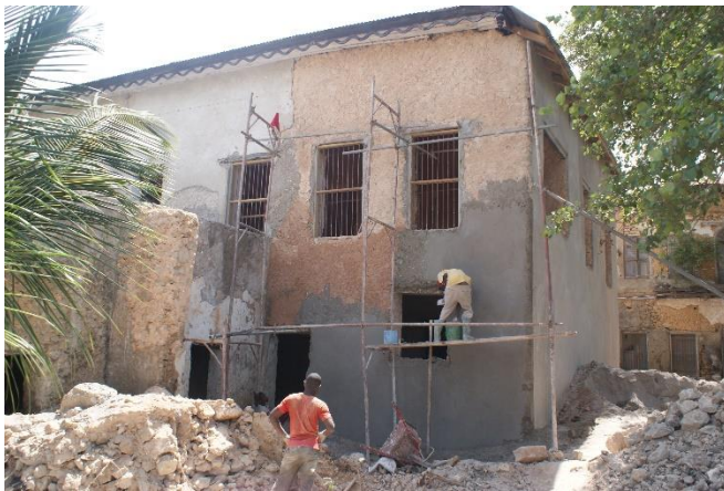
Fig 25: Firefly lounge during restoration
