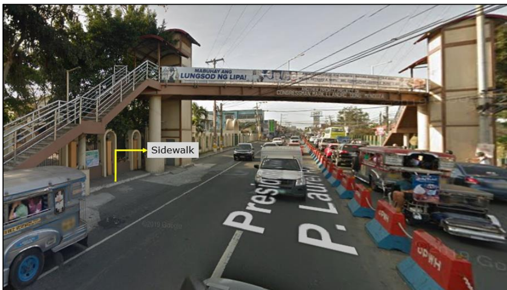
FIGURE 24. Grade-separated facility that obstructed the sidewalk (Google Maps, 2020b)
