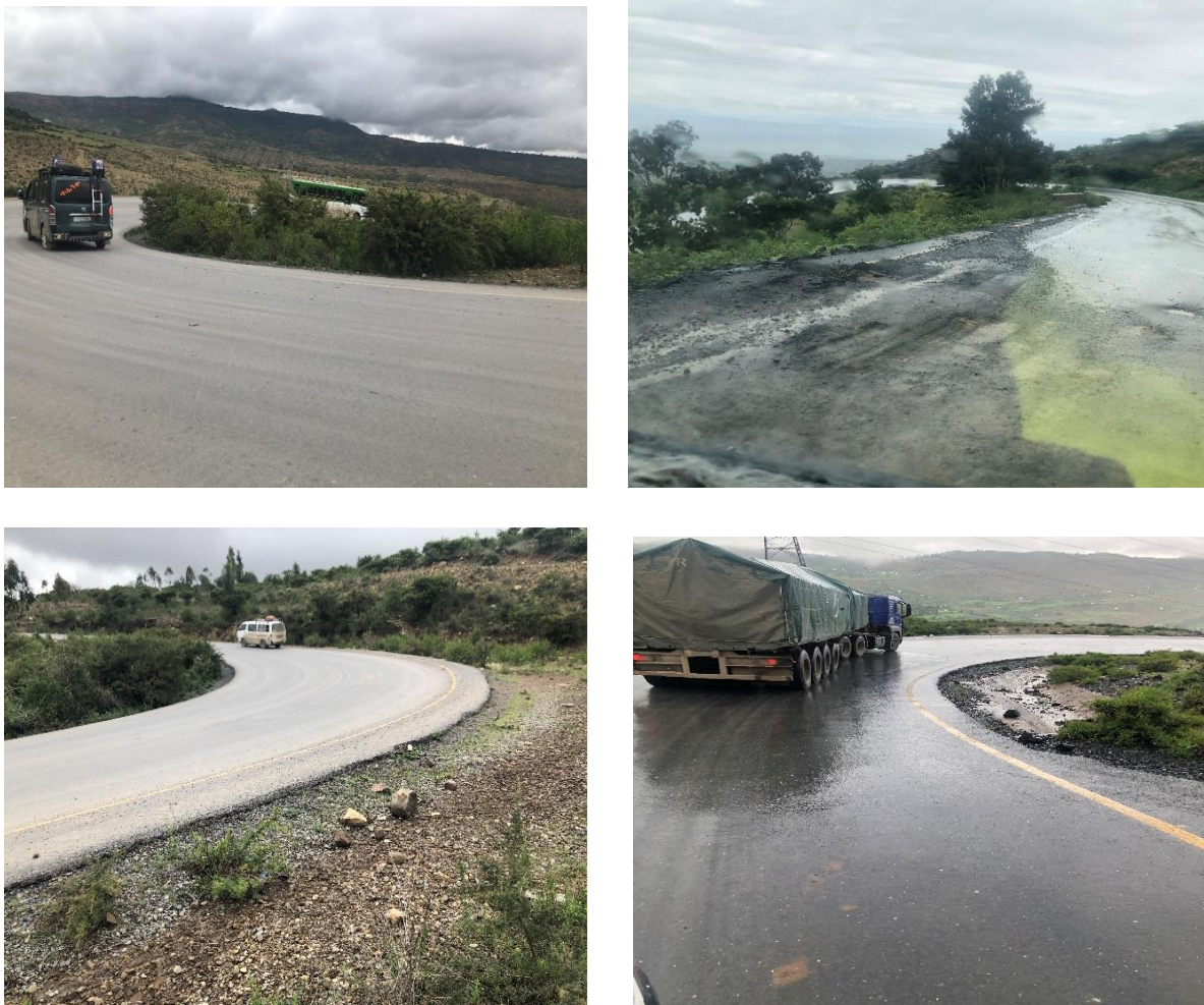
Figure 9: Some features of Simret district road section (Researcher)
