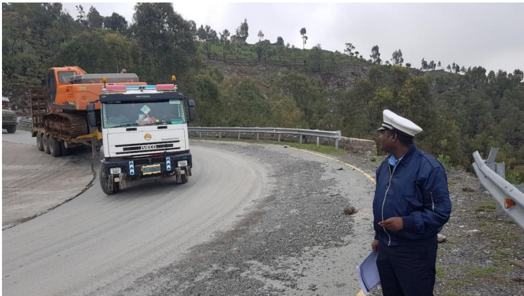
FIGURE 19 Horizontal curve in route from Wukro -Adi-Abaggi that experienced higher traffic crash records (taken by the researcher during site visit).
