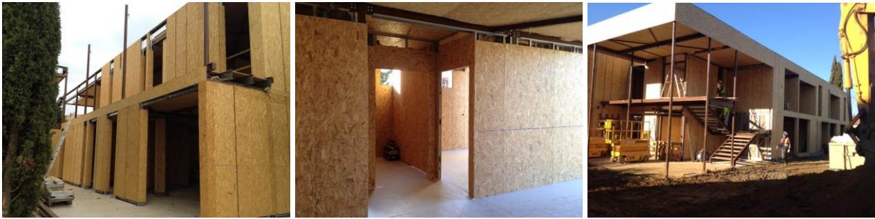
Fig. 2: Erection of CAP Solidarité building – La Croix Valmer, France
