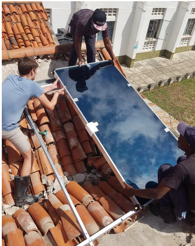
Figure 60: Installation of the first panel
