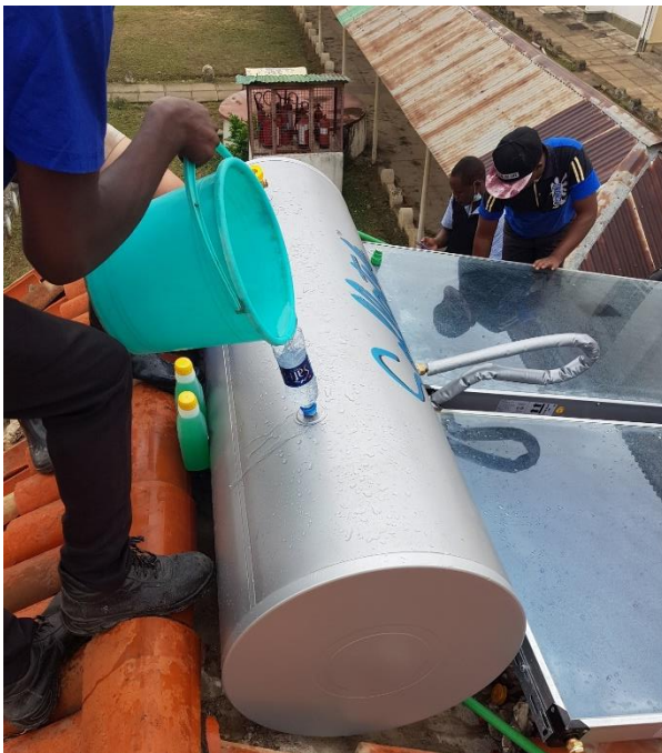
Figure 66: Filling the inner tubing with water (A), adding glycol to the water (B)
