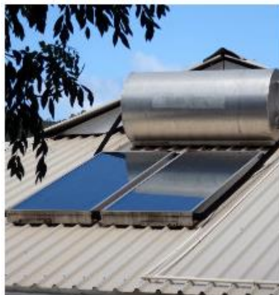
Figure 16: Storage tank placed on the sloping roof [26]
