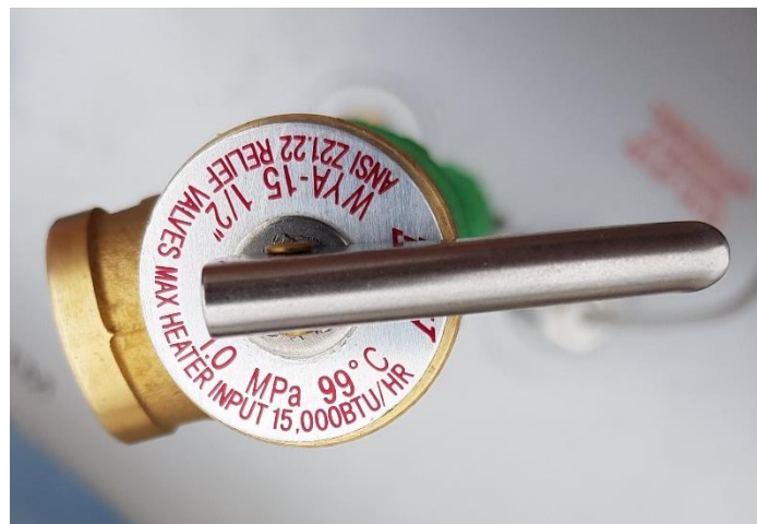
Figure 77: Details pressure release valve
