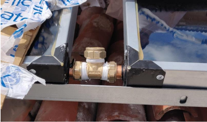
Figure 63: The T-connection between the inner tubes
