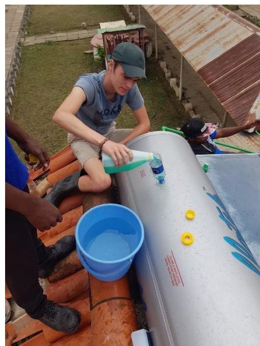
Figure 66: Filling the inner tubing with water (A), adding glycol to the water (B)
