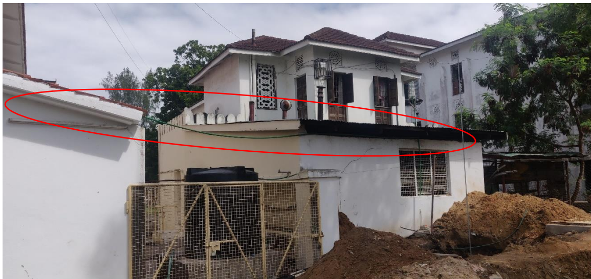
Figure 74: Further progression of the hot water pipe
