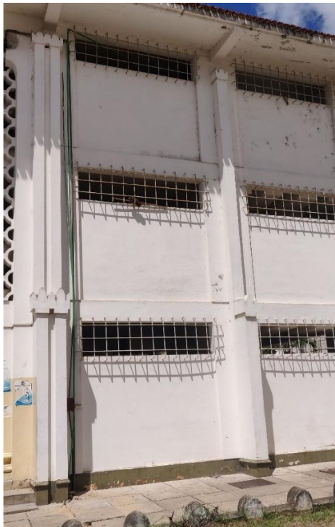
Figure 71: Cold-water pipe lead to the ground
