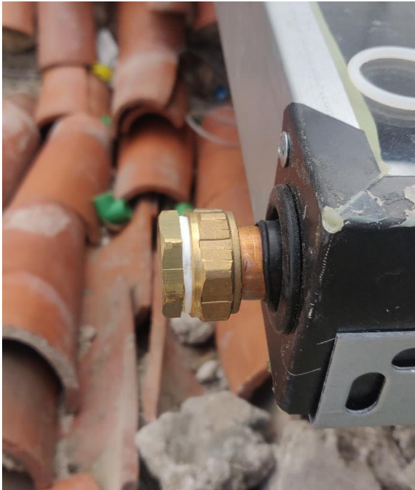
Figure 62: Caps on the end of the inner tubing
