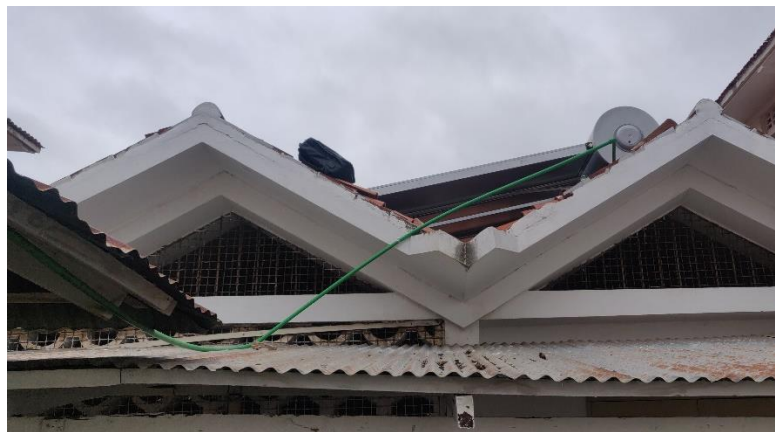
Figure 72: Cold-water pipe under the small roof (A), connected to the storage vessel (B)
