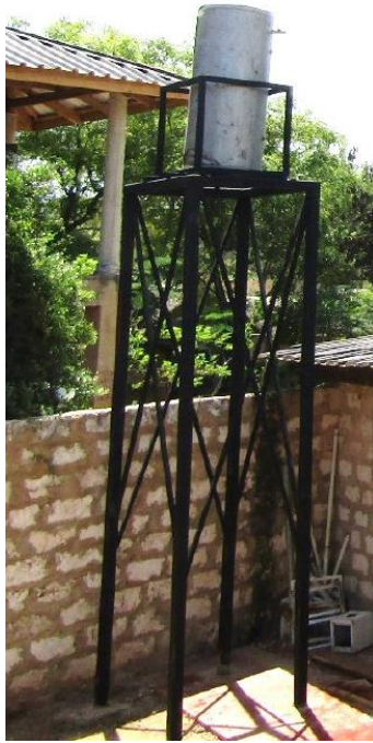
Figure 47: Steel construction for the water storage tank [2]
