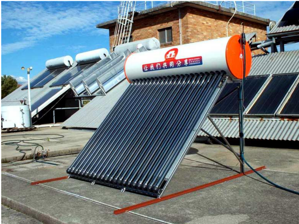
Figure 24: Example evacuated tube solar collector [30]
