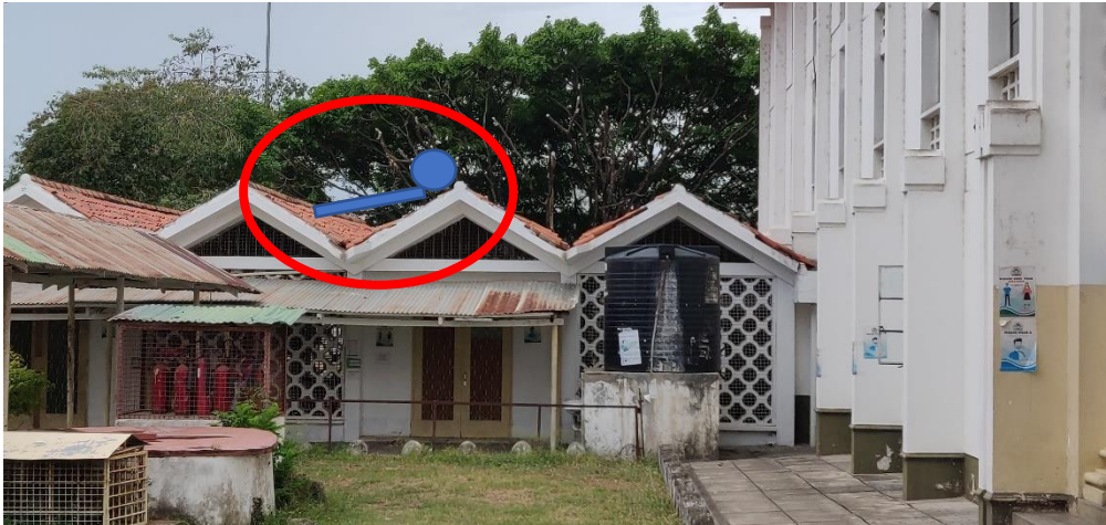
Figure 55: The sloping roof for the solar collector
