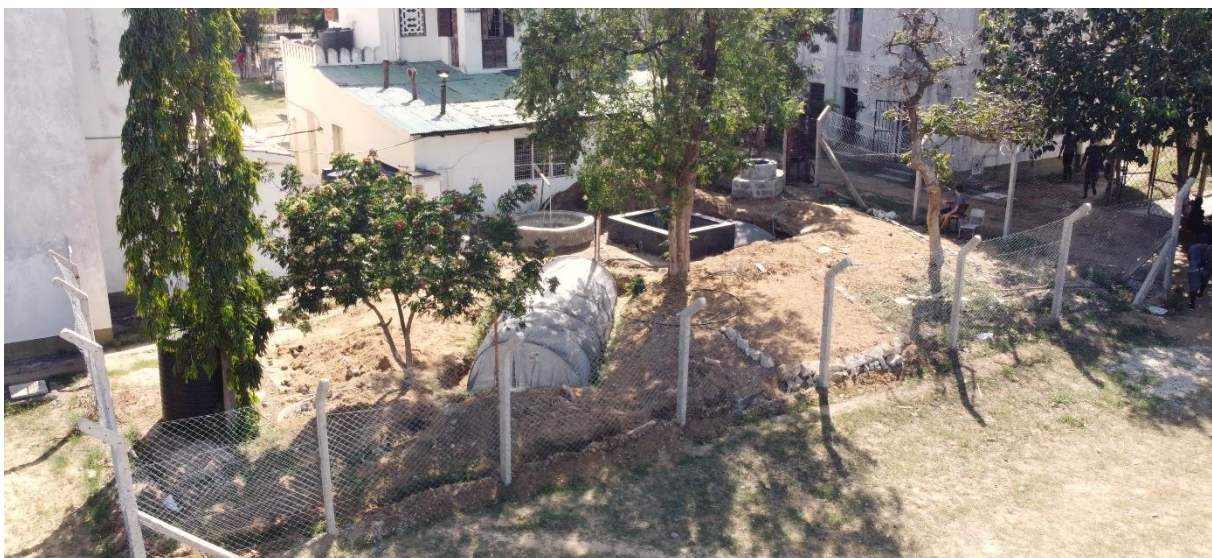
Figure 11-8: Status of the project on May 17, 2021
