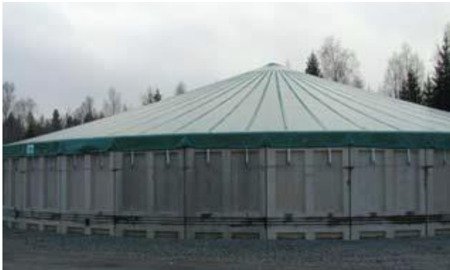
Figure 6-5: Large scale digestate tank with a cover [31]
