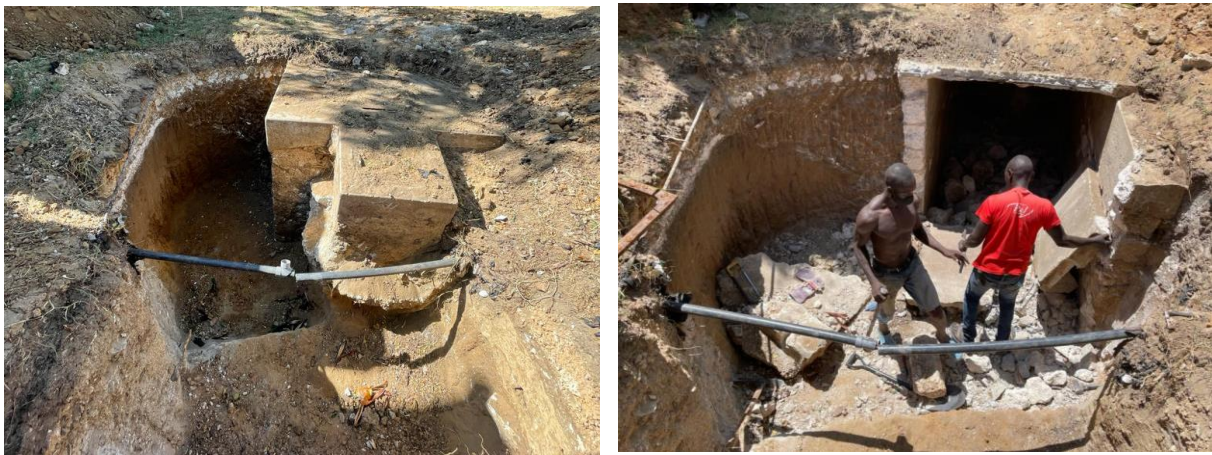
Figure 10-1: Removal of the septic tank and the piping
