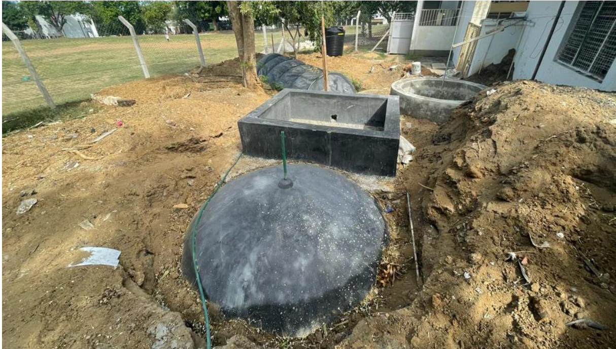
Figure 10-7: Status of the project on May 17, 2021
