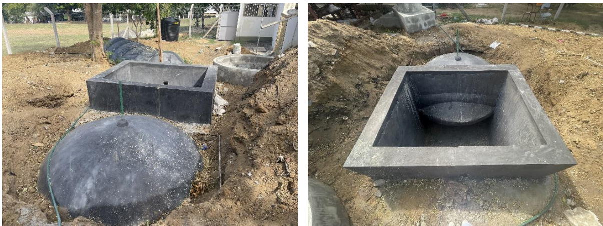
Figure 11-3: Fixed-dome installation
