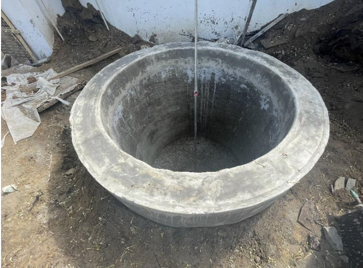
Figure 11-5: Outer cylinder of the gasholder
