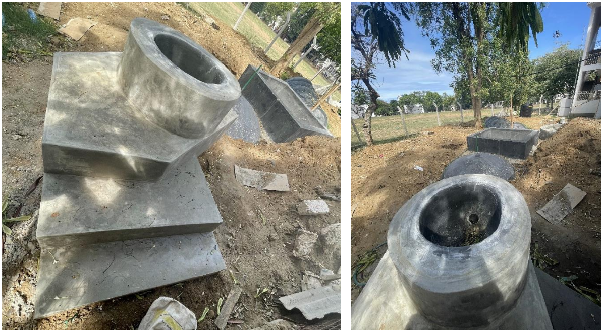
Figure 11-1: Inlet reservoir
