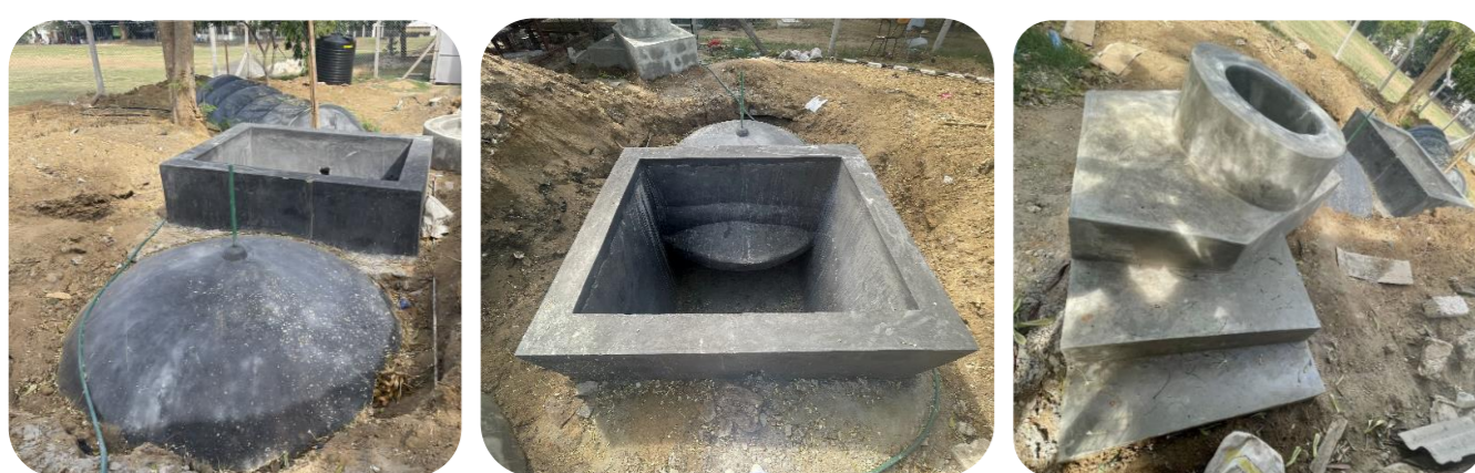
Figure 3: Fixed-dome digester, overflow tank and inlet reservoir
