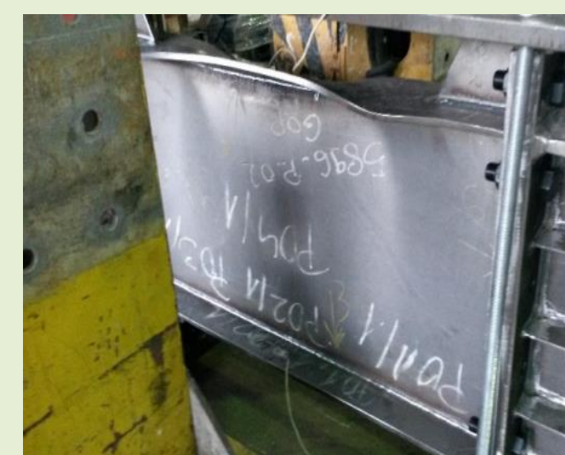
Fig. 8: Unstiffened damaged girder
