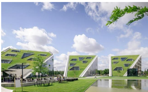
Figure 5: Extensive green roof (Corda Campus, Hasselt), by Ecoworks
