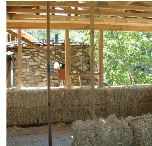
Figuur 13: Post-and-beam methode (Ruppert, 2014)
