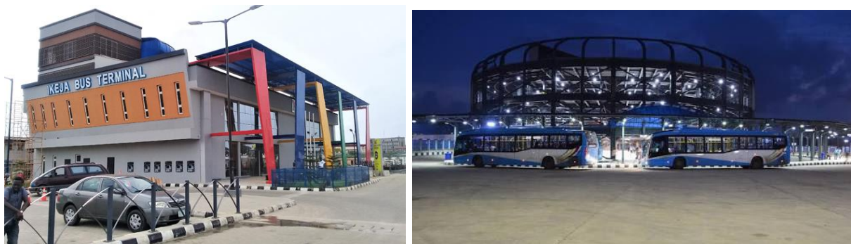
FIGURE 10 Ikeja Bus terminal and Oshodi Intercity Terminal 3 (ecogreennews.com).
