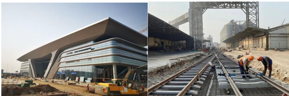
FIGURE 12 Apapa Port railway under construction (Chigozie, 2021).
