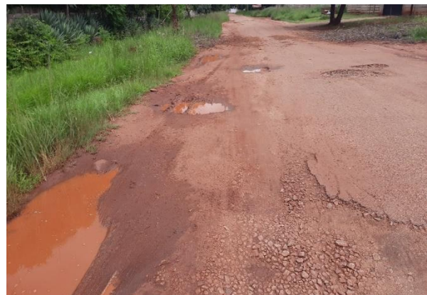
Potholes filled with water
