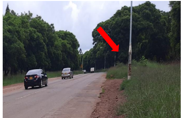
Poor sight distance Access road (Snowdon) blocked by vegetation
