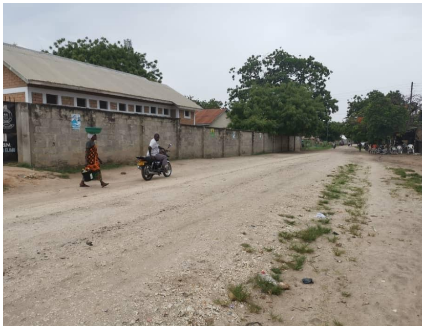
FIGURE 3 The unpaved urban road alongside Kivukoni Primary School on the left.
