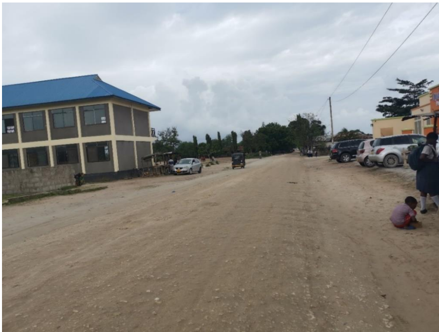
FIGURE 1 The unpaved urban road alongside Ufukoni and Kigamboni Primary Schools.
