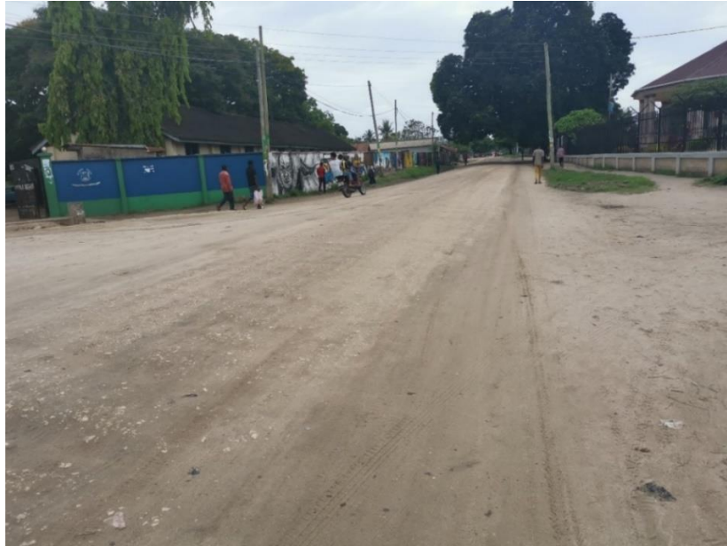
FIGURE 2 The unpaved urban road alongside Kigamboni Primary school on the left.
