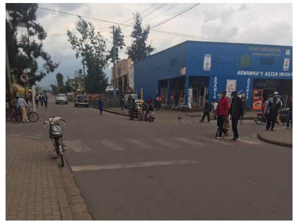
FIGURE 3 Concrete pavers elevated sidewalk
