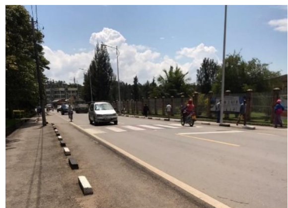
FIGURE 7 curb separated sidewalk
