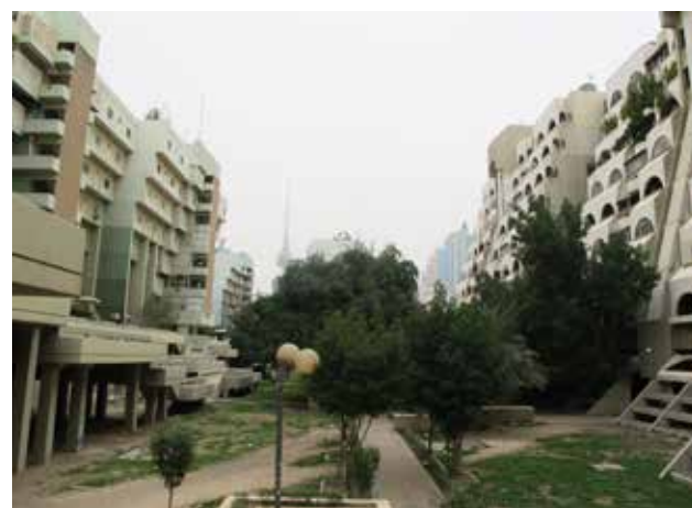
[9] The open green spaces in-between the buildings of the Al Sawaber Complex in Kuwait in their current condition (2019). The public character of the ground floor is perceived through the columns, as they form a shaded walkway.
