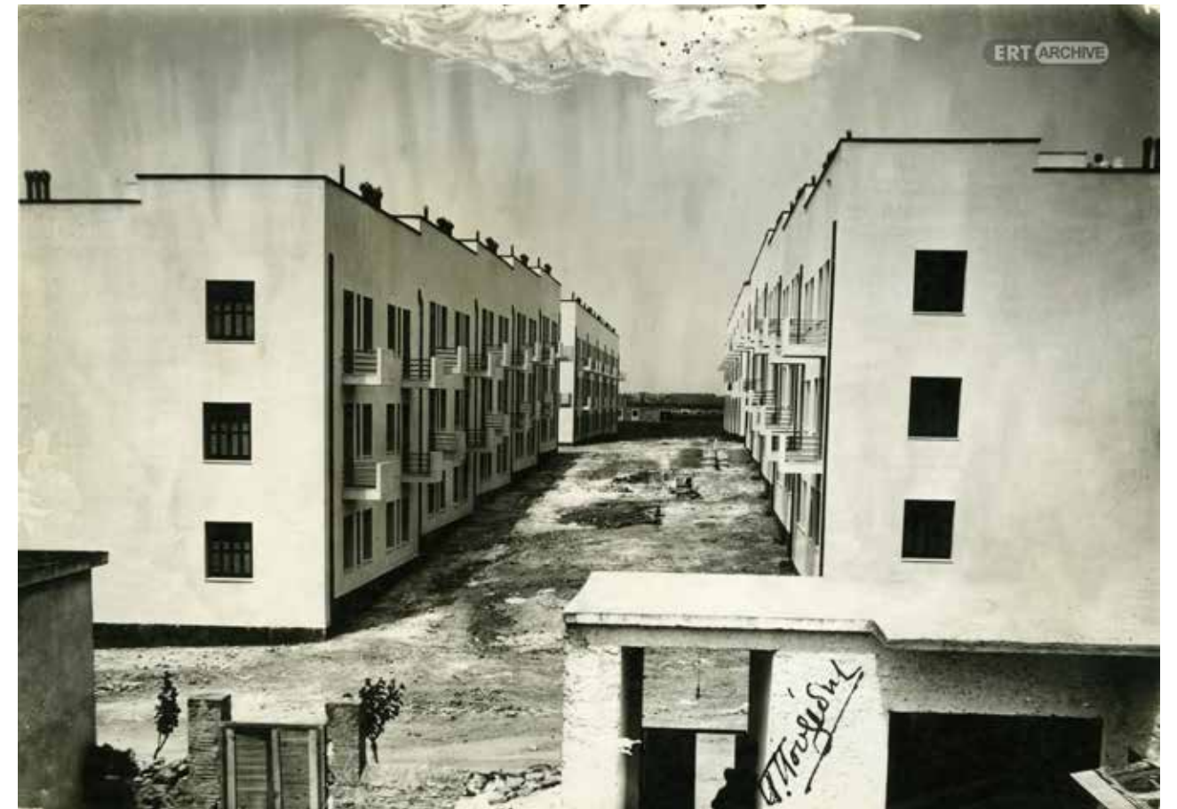
[1] This image of the refugee housing at Prosfygika in Athens is taken shortly after completion (1936). The dire circumstances of the urgent need for housing can be deduced from this image. The buildings were set up in a short matter of time due to extensive prefabrication and standardisation.
