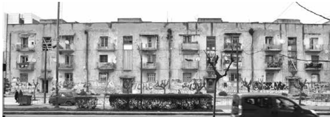
[5] Inspired by the image of Quartiers Modernes Frugès in Pessac [4], Papageorgiou, A. (2019) took a picture of the façade of the Prosfygika housing project in Athens (2019), in which the vernacular adaptations (such as conversions of windows, the transformation of balconies, making versus removal of openings, and the addition of sunshades) appear.
