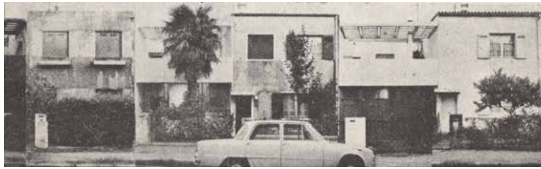
[4] On the different elevations of the buildings of Quartiers Modernes Frugès by Le Corbusier in Pessac (Boudon, 1972), the vernacular adaptations of the inhabitants (such as shutters, coverings, different colours) can be deduced from the image.
